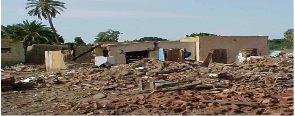
Photo shows damaged Buildings
